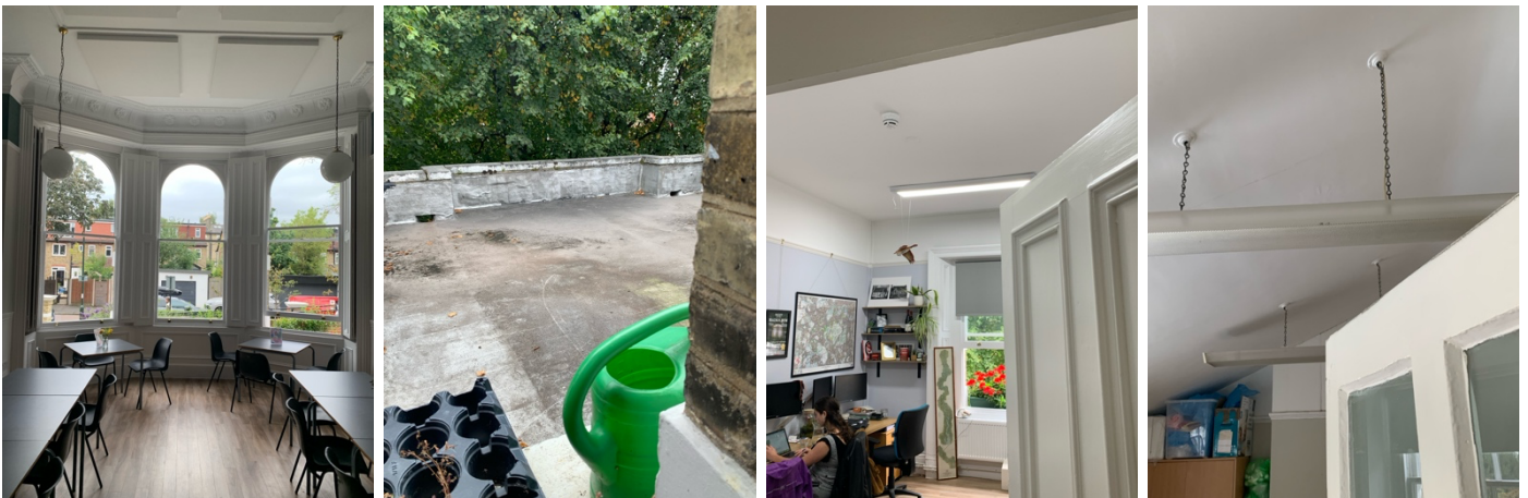
Figure 1: (A) Double-glazed windows throughout the building (B) Poorly-insulated flat roof over the hall. (C) LED light fittings. (D) Old, fluorescent lighting.
