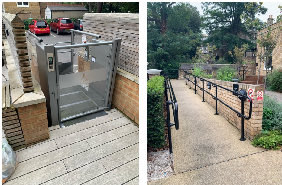
Figure 5: (A) Passenger lift to the back of the building to allow disability access to the parking lot. (B) Accessibly ramp at the front of the property.
